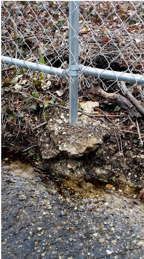
Cement pilings in stream and stream bed.
