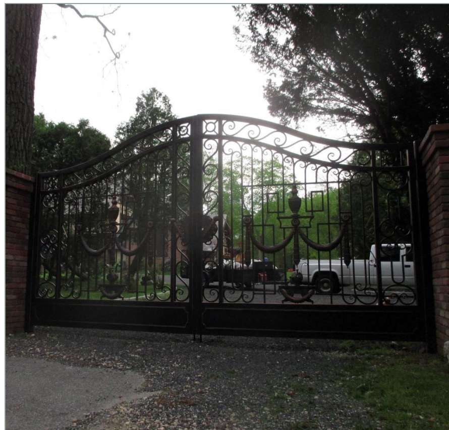
Non-confirming iron gates, 156 Cove Road
