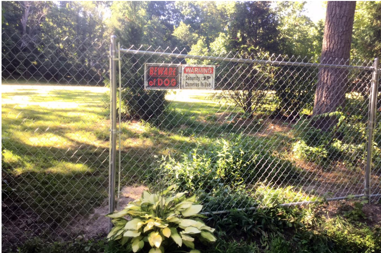
Fence installations commenced Saturday, August 6, 2016 (photo by E. O'Neill)
